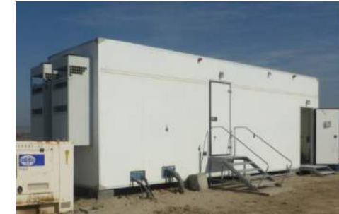
CTC Shelter installation
